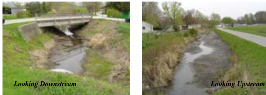
Figure 7-4. Oliphant Ditch at College Avenue
